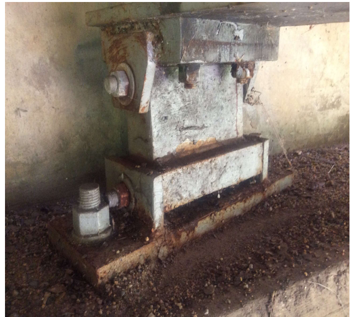
PHOTO 2 Description End bent bearing rust Bearing #4,5,6,7
