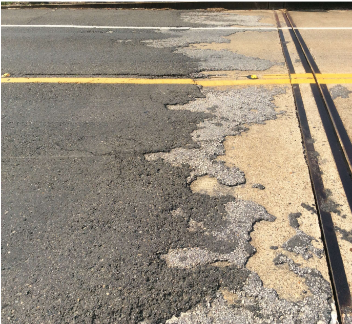
PHOTO 1 Description ASPHALT ON APPROACH COMING APPART END BRIDGE
