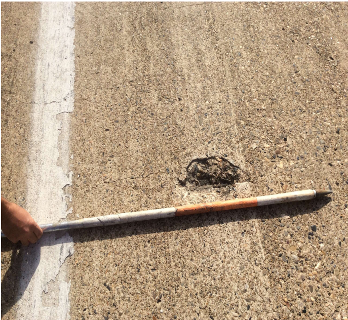
PHOTO 4 Description Spall in deck with rebar exposed span 1..
