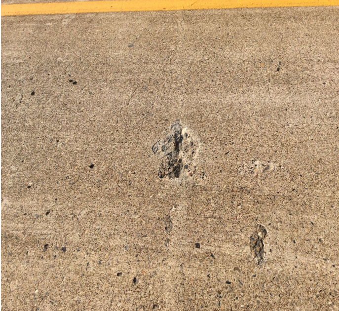
PHOTO 3 Description DECK SPALL SPAN 2 LEFT SIDE
