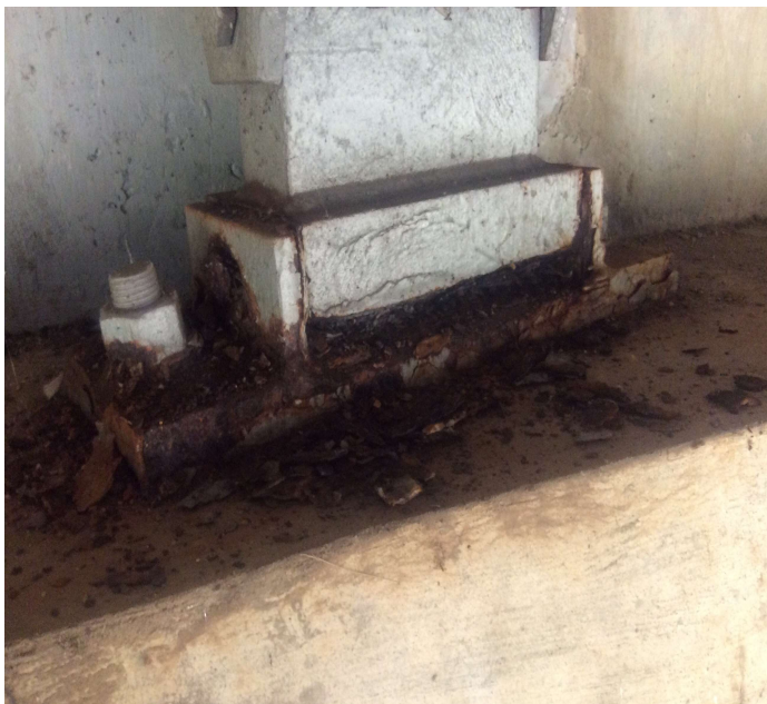
PHOTO 3 Description Bent 1 bearing #3 rust and section loss
