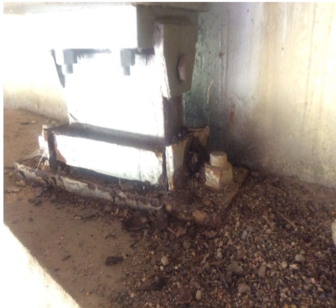
PHOTO 1 Description Bent 1 bearing rust, ears on bearing broke photo of bearing 4
