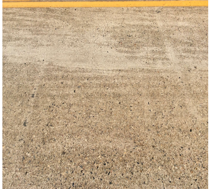
PHOTO 5 Description Sealable deck cracks and map like cracking. Photo taken of span 2
